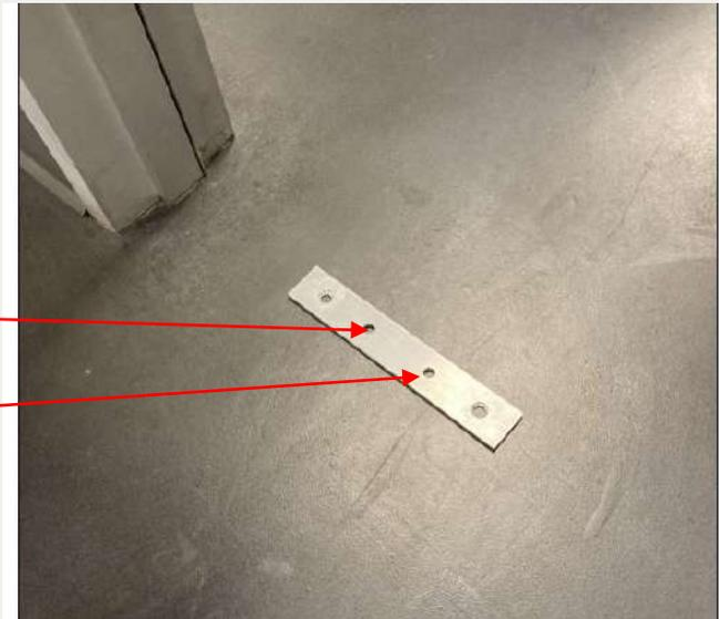
NOTE: Apply ample amount of silicone under the sill as part of installation.
