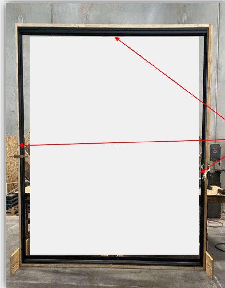
**A** Secure the Door Frame with screws into the Rough Opening through each pre-drilled hole in each Jamb and the Head of the frame
